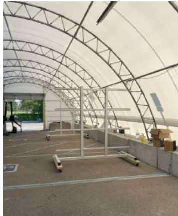
Large shell winter storage, summer workout facility $62,000
